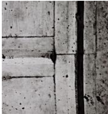
Figures 6 et 7 : Joints en V du béton Photos issues de ROSELLINI, Anna. Louis Kahn towards the zero degree of concrete 1960-1974. EPFL Press, 2014. p. 58-59. Treatise on Concrete .
