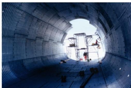
Construction of Halley III, showing interior of the Armco steel tube in which the new station buildings would be housed, 1973 (Archives ref: AD6/19/3/C/Z38). Photographer: Vivian Fuchs (Director, FIDS)
