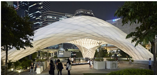
Figure 2. The 'ZCB Bamboo Pavilion' during a night time event Source: Chinese University of Hong Kong's School of Architecture
